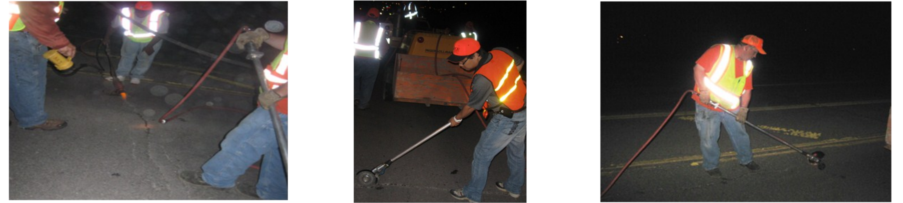
NDOR crews using a conventional hot air blaster (left) and the new device (middle and right)
