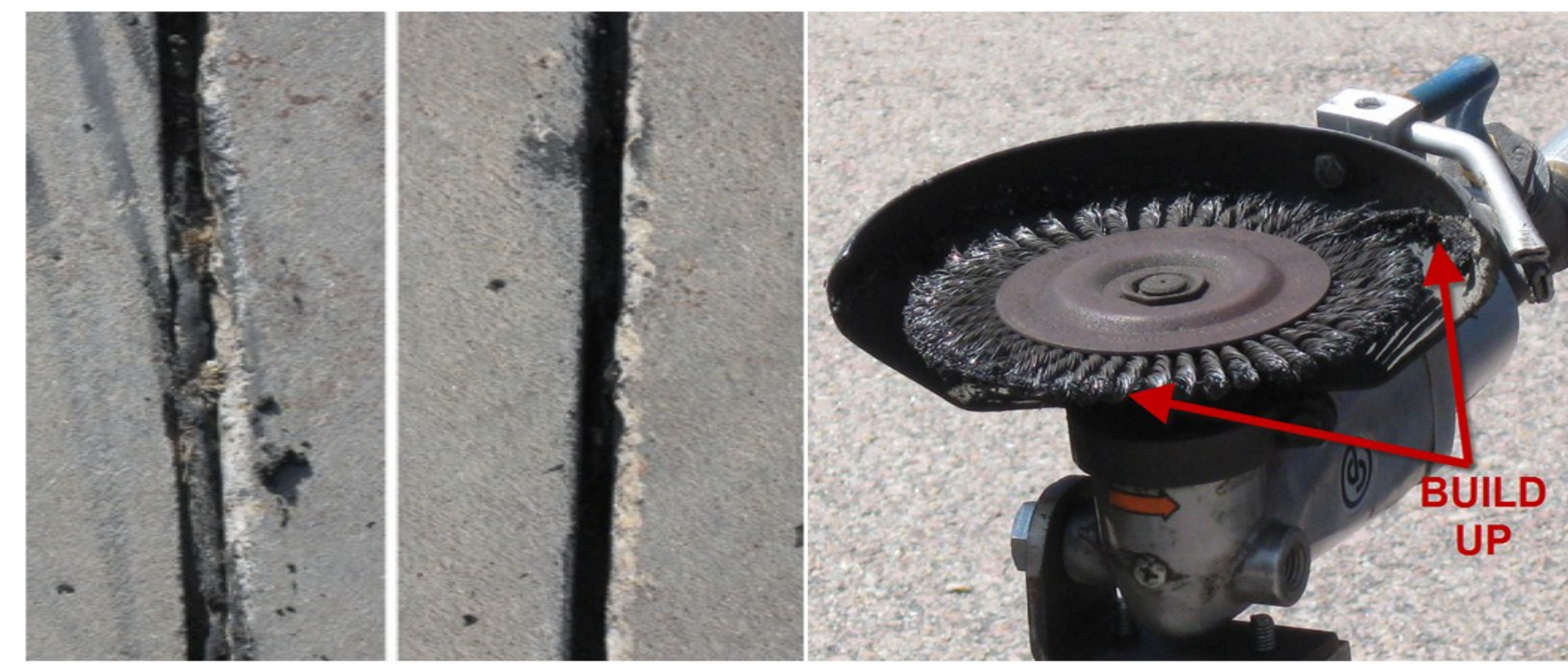
Effective preparation of previously sealed crack, with sealant residue buildup being shown on the device
